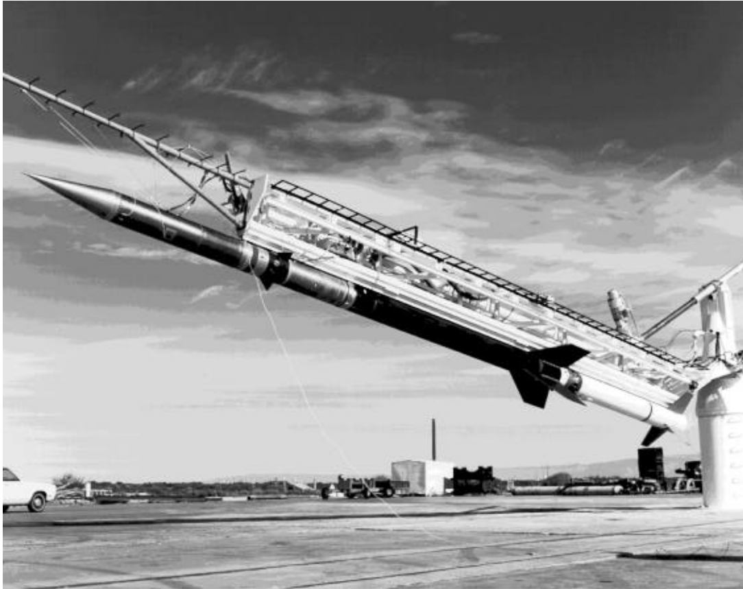
Figure E-19. Terrier-Black Brant VC Launch Vehicle
